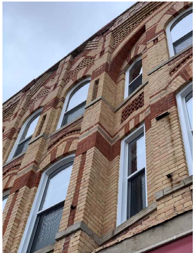
06_29 Sykes_Heritage Facade Detail
