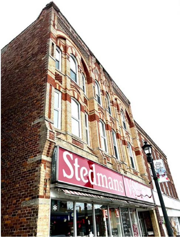
03_29 Sykes_Heritage Facade Detail
