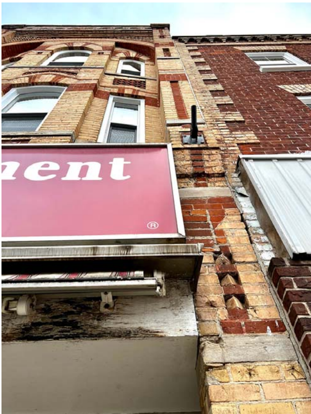
05_29 Sykes_Heritage Facade Detail
