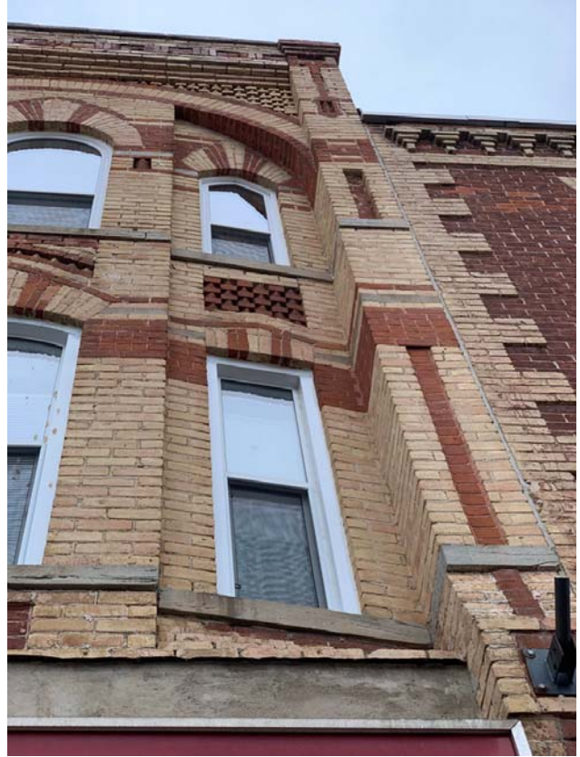
04_29 Sykes_Heritage Facade Detail
