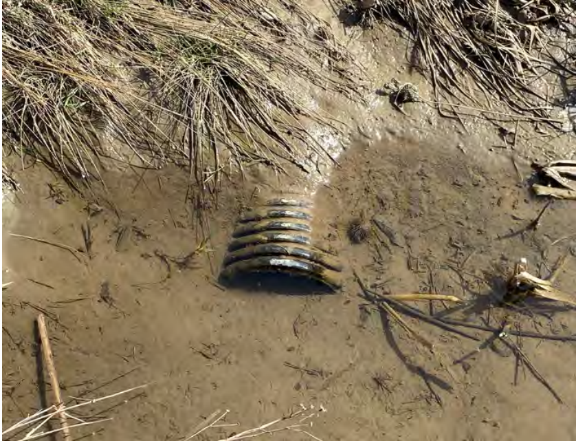
Figure 2 - Existing Tile Outlet at Northwest Corner of Lot 28, Concession 3
