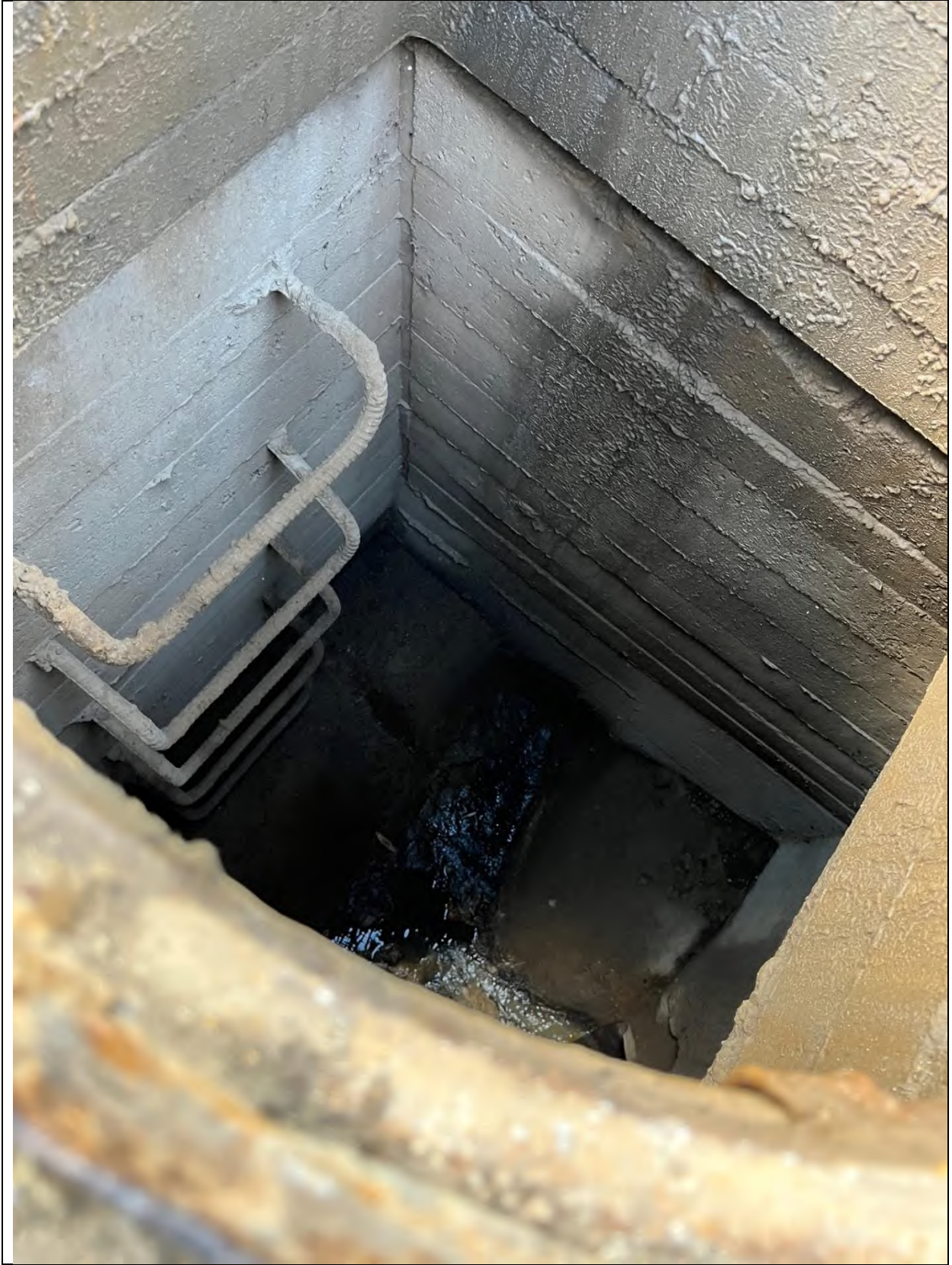
Outlet 3 Maintenance Hole
