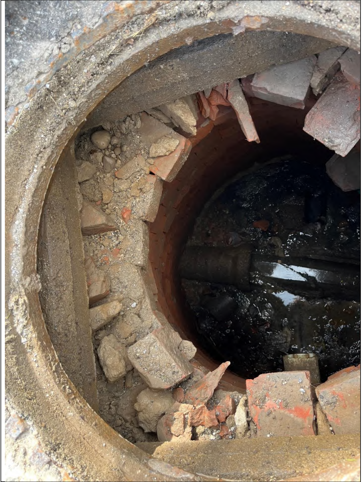
Outlet 2 Maintenance hole
