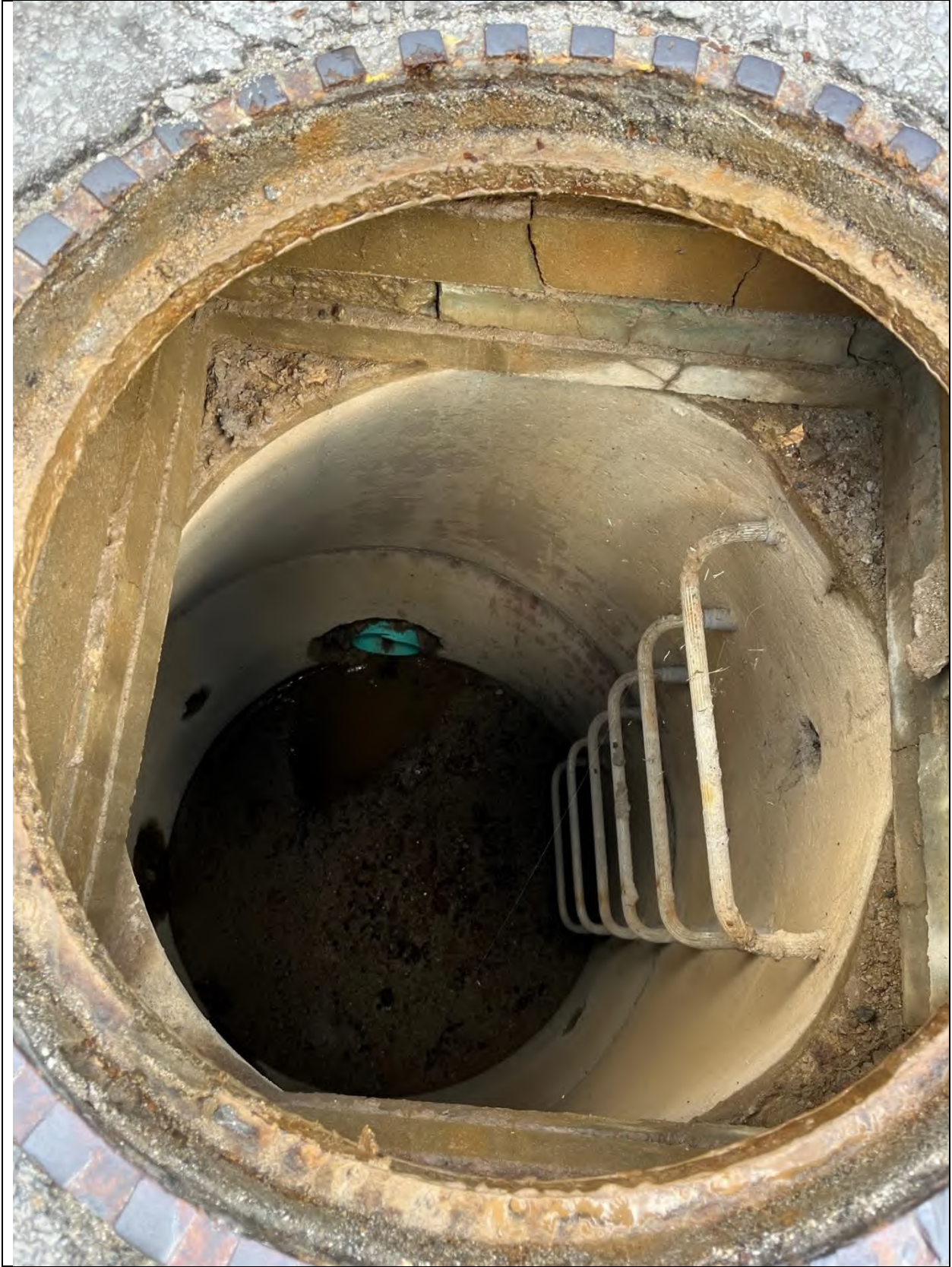
Outlet 1 Maintenance hole
