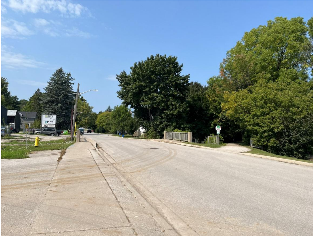
Figure 28: Edwin Street East, looking northwest. The subject bridge and Georgian Trail are visible to the right of the roadway (A.S.I., 2024).
