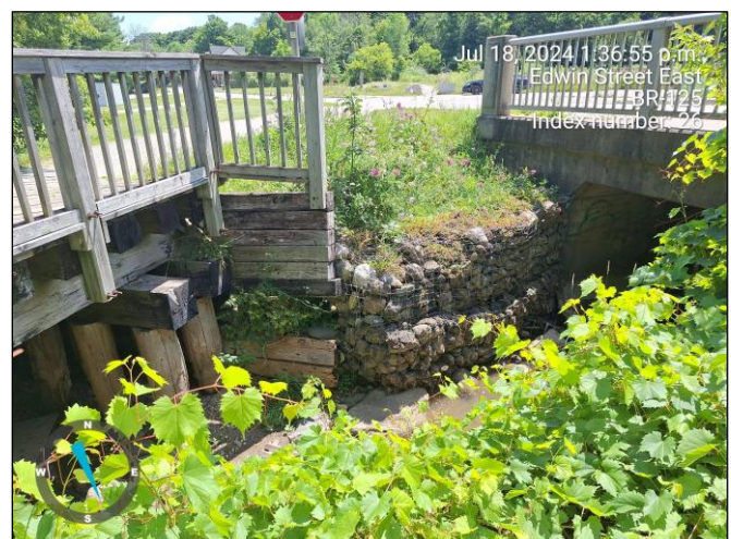
Image A6 – Gabion baskets at southwest corner.
