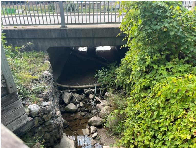
Figure 23: Meaford Creek, looking south from the subject bridge toward the Edwin Street East culvert (A.S.I., 2024).
