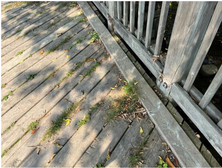
Figure 11: Detail view of the bridge deck and timber curb (A.S.I., 2024).
