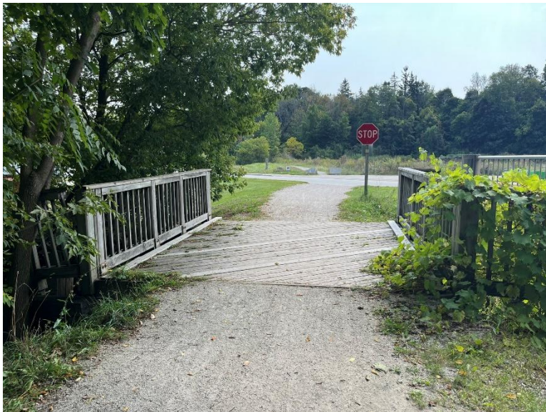
Figure 10: The timber bridge deck, looking southeast (A.S.I., 2024).
