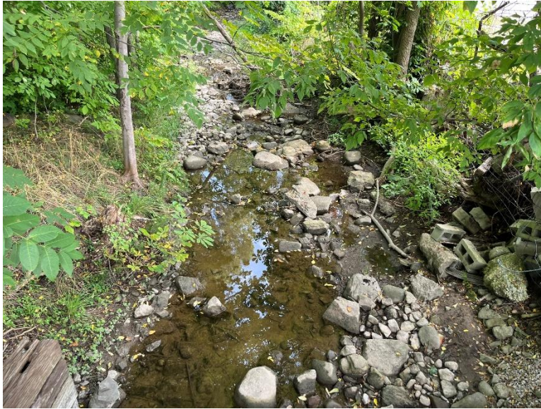
Figure 22: Meaford Creek, looking north from the subject bridge (A.S.I., 2024).
