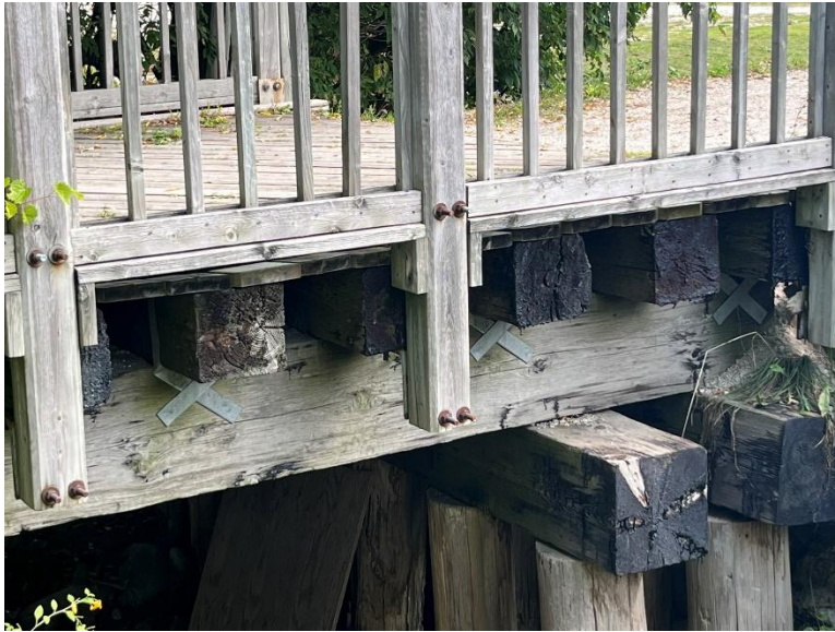
Figure 3: The bridge superstructure, the beams and railroad ties are visible beneath the railing (A.S.I., 2024)
