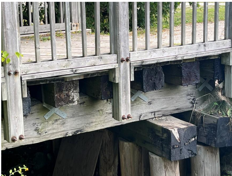
Figure 11: The bridge superstructure, the beams and railroad ties are visible beneath the railing (A.S.I., 2024)
