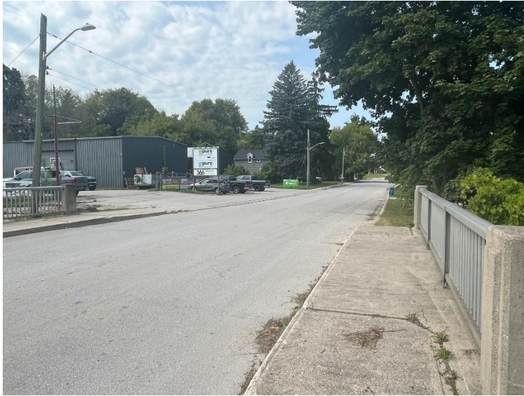
Figure 26: Looking northwest from the Edwin Street East culvert. The industrial property on the south side of the street is visible on the left and residential properties are visible in the distance (A.S.I., 2024).
