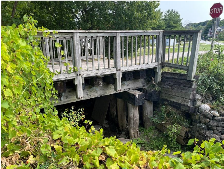
Figure 10: South elevation of the subject bridge, looking northeast (A.S.I., 2024)
