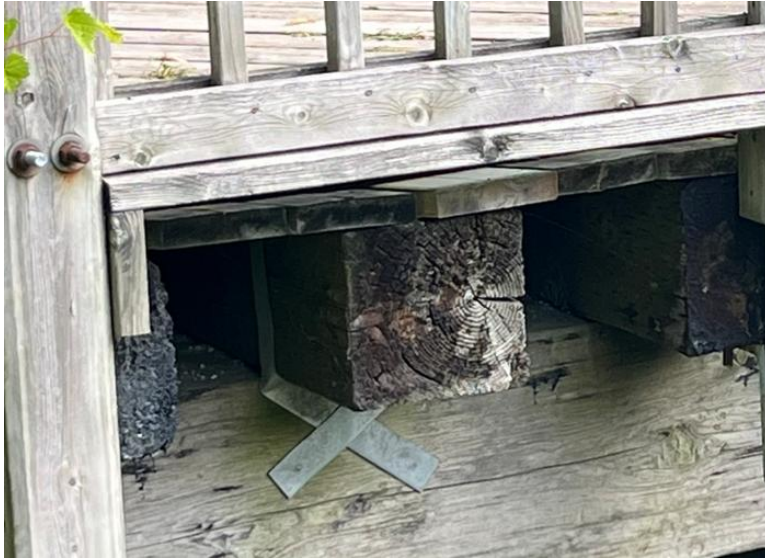
Figure 12: Detail view of the strapping connecting railroad ties to beams (A.S.I., 2024)
