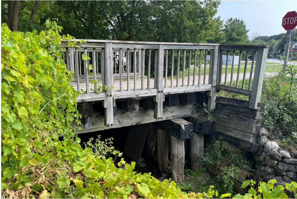
Figure 2: South elevation of Meaford Bridge No. 125, looking northeast (A.S.I., 2024)
