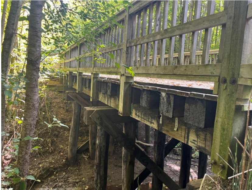
Figure 30: The comparable bridge on the Georgian Trail between Montgomery Street and Swarthmore Drive (A.S.I., 2024).
