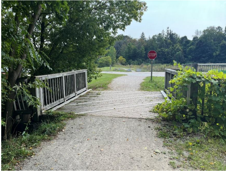
Figure 18: The timber bridge deck, looking southeast (A.S.I., 2024).
