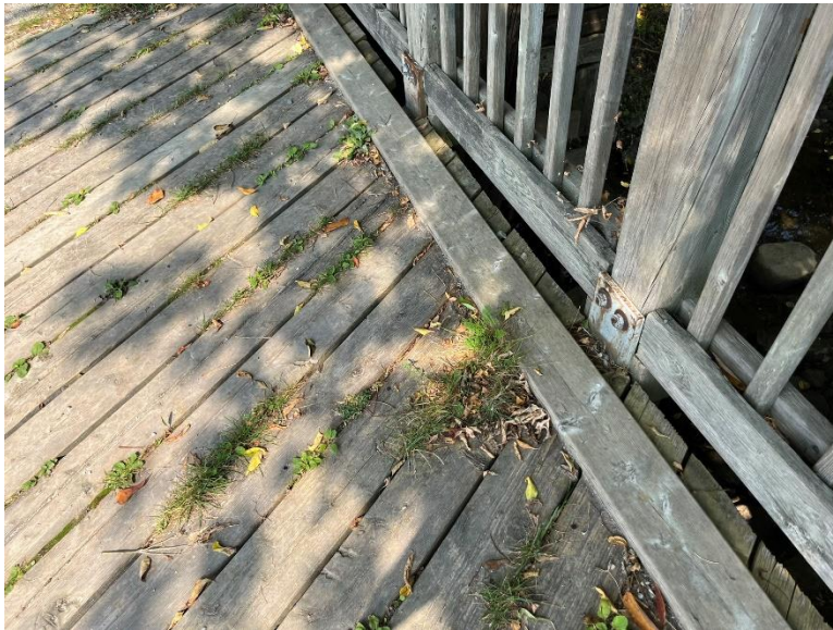
Figure 19: Detail view of the bridge deck and timber curb (A.S.I., 2024).
