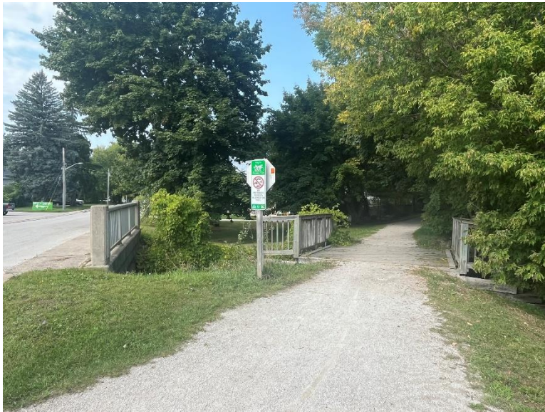
Figure 25: The Georgian Trail over the subject bridge, looking northwest. Edwin Street is on the left (A.S.I., 2024).
