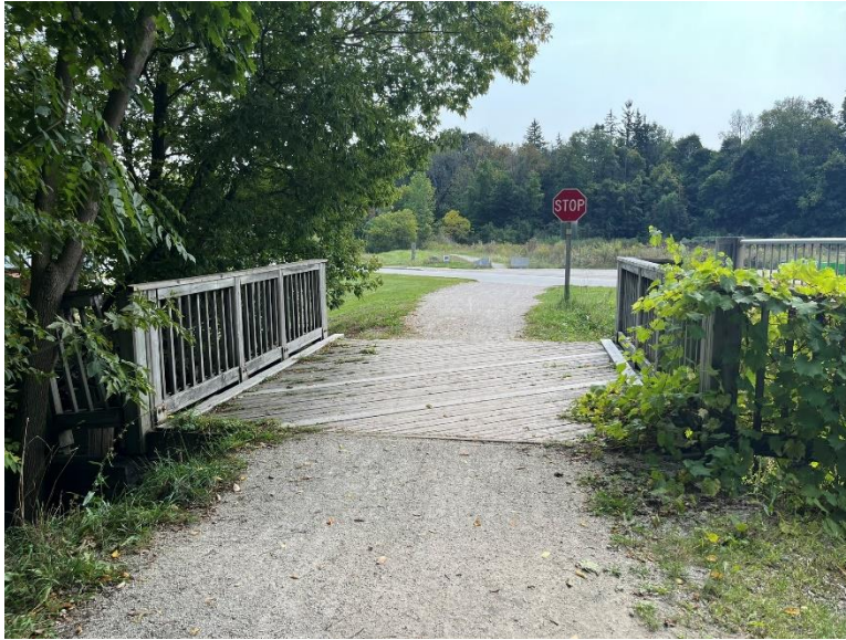
Figure 18: The timber bridge deck, looking southeast (A.S.I., 2024).
