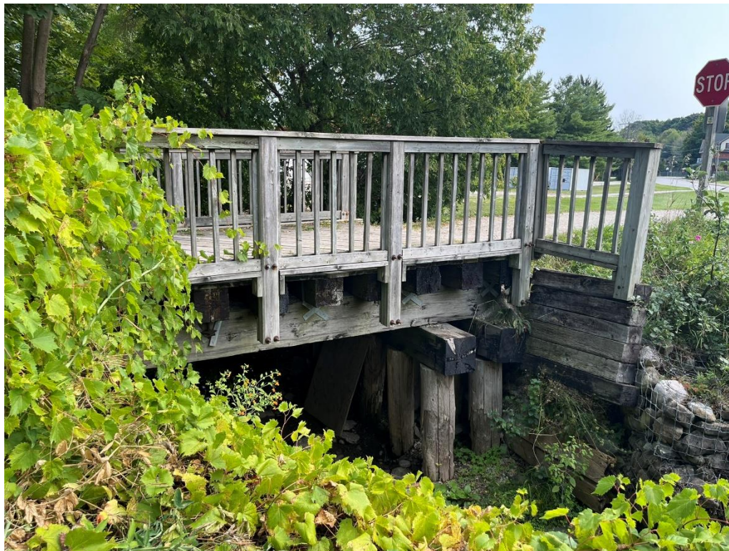
Figure 2: South elevation of Meaford Bridge No. 125, looking northeast (A.S.I., 2024)
