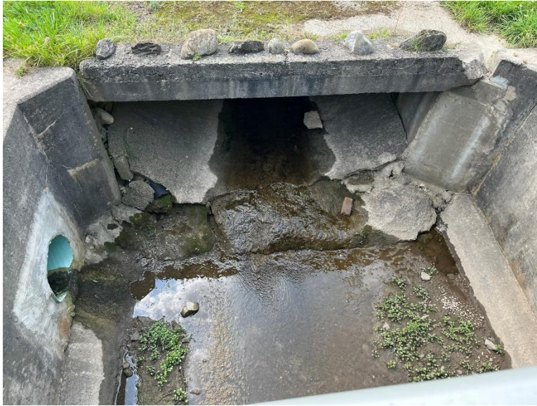
Figure 24: The culvert on the south side of Edwin Street East, looking south (A.S.I., 2024).
