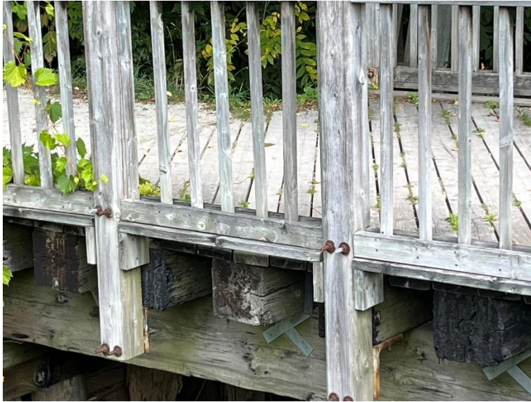
Figure 20: Detail view of the railing system on the southern elevation. Note the bolts connecting the railing to the superstructure (A.S.I., 2024).
