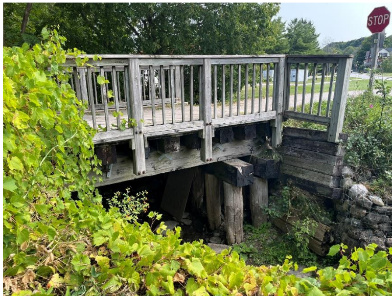
Figure 2: South elevation of the subject bridge, looking northeast (A.S.I., 2024)
