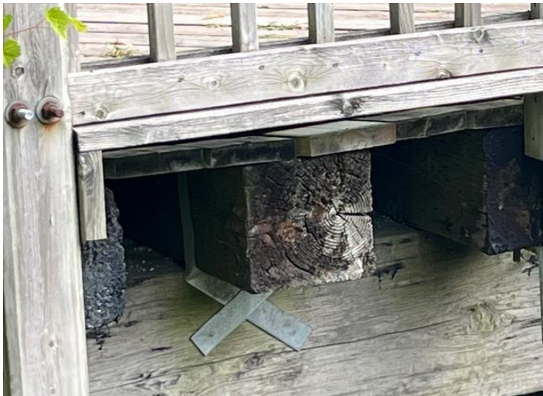
Figure 4: Detail view of the strapping connecting railroad ties to beams (A.S.I., 2024)
