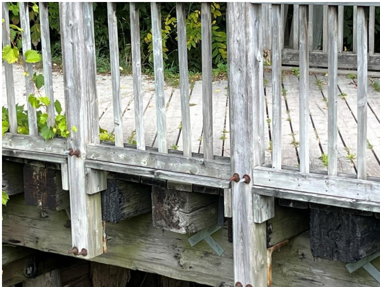
Figure 12: Detail view of the railing system on the southern elevation. Note the bolts connecting the railing to the superstructure (A.S.I., 2024).
