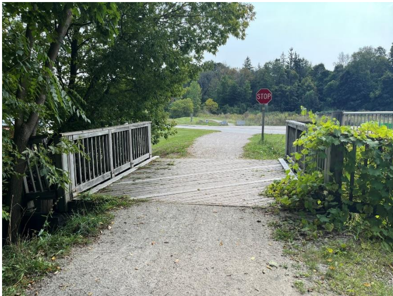
Figure 10: The timber bridge deck, looking southeast (A.S.I., 2024).
